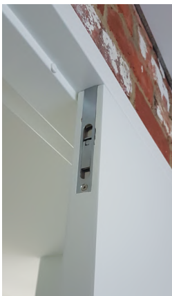
25 DOOR BOLTS & PRIVACY HARDWARE
